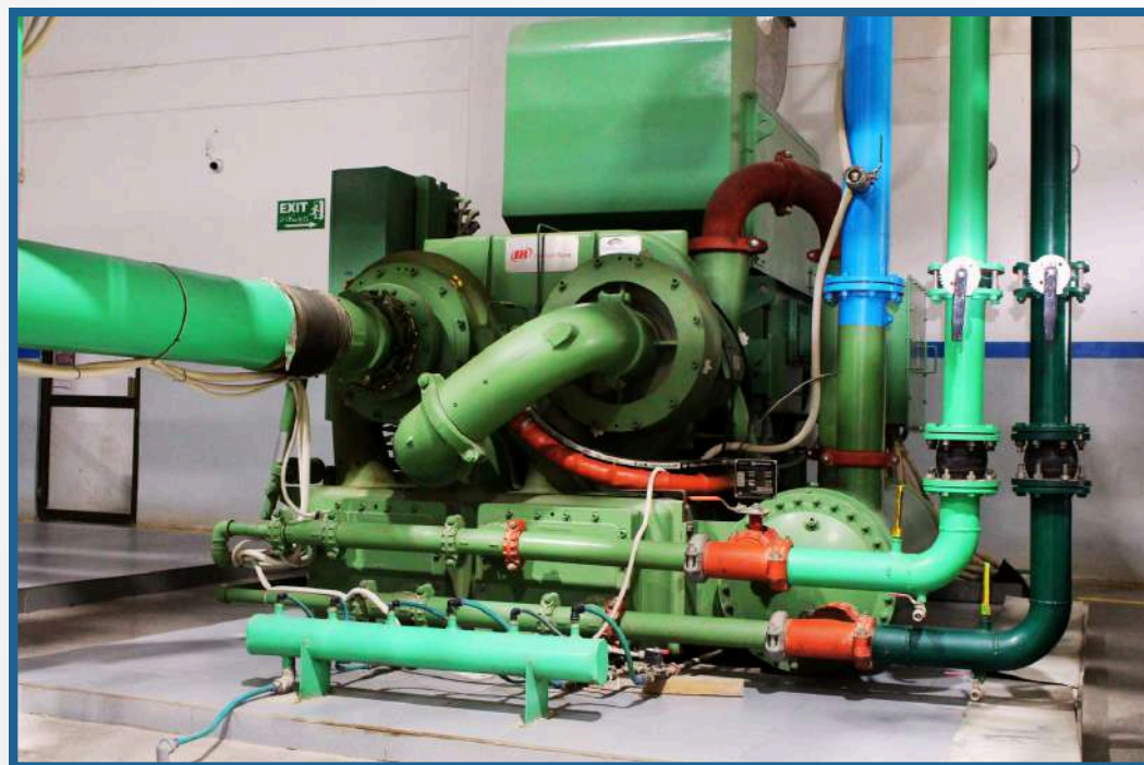
INGERSOLL RAND Compressor TA 6000 (670 KW)
